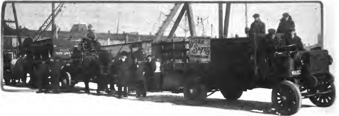
American La-France truck equipped with hydraulic transmission hauling a 45-ton load consisting of a frame for the door of the new vaults of the Bank Clearing House in New York City. The frame was placed upon a four-wheel wagon which, empty, weighed 16,400 pounds. The door frame weighed 52,600 pounds. The truck was loaded with five steel plates for the vault which weighed 12,100 pounds. The truck itself weighed 9,000 pounds, so that the total load to be moved was 90,000 pounds.
